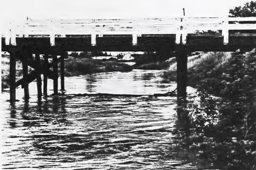
u/s side of bridge HWM VR 83-3 26 June 1983
